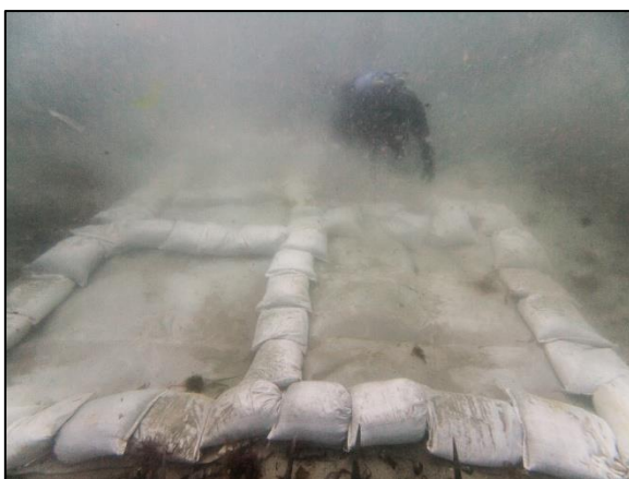
Fig 10 - Terram and sandbags one day after installation over the site of the small excavation in June 2012
