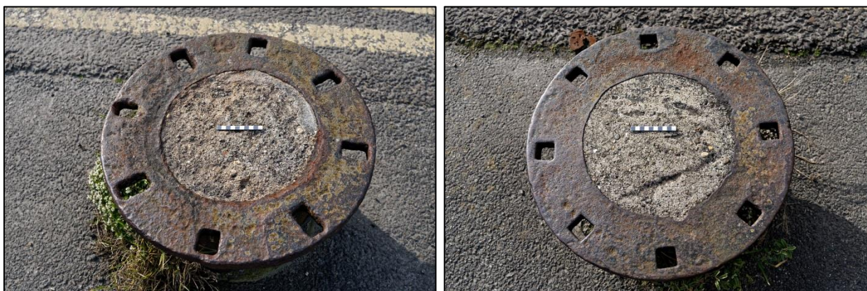
Fig 38 - Examples of rectangular and square flange bolt holes – these are 13 inch rising mains reused as mooring posts at Penzance quay (internally filled with concrete). The scale is 10cm long.
