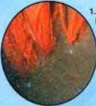
1. Initial sediment build-up covering mattress and the foot of the fronds.
