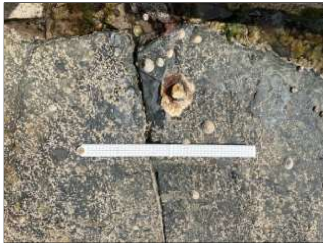
Fig 35: Traces of the ARC scaffold; part of a steel tube cemented into the rocks
